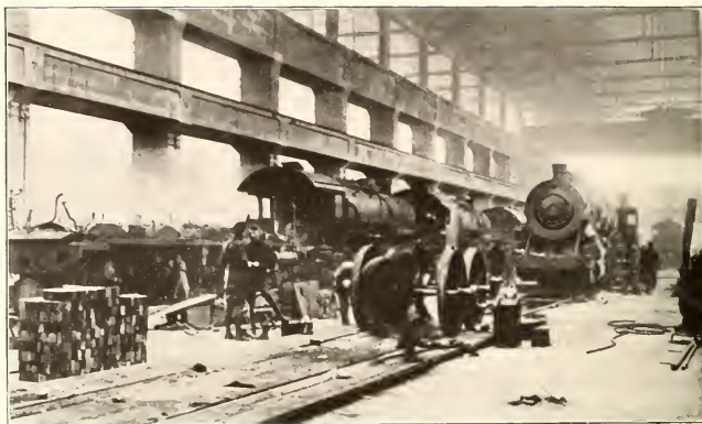
INTERIOR OF THE RAILROAD REPAIR SHOPS AT NEVERS, WHICH WERE DIRECTED BY CHARLES S. GASKILL, '99
